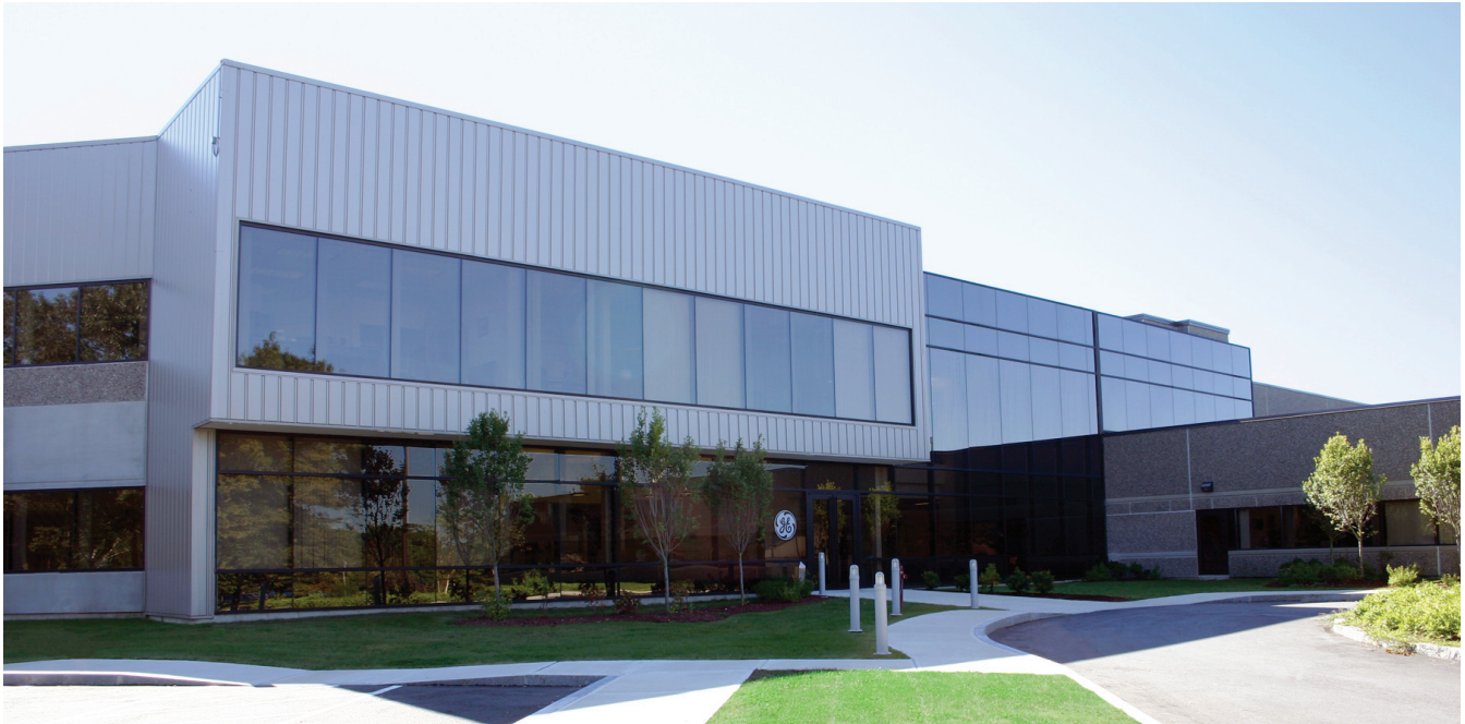
GE Sensing & Inspection Technologies building in Billerica, USA
